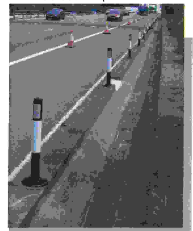
6. Take NF Verge Marker and push down firmly making the mound of glue go up inside the middle of the pole cones and spread across to whole base of product.
