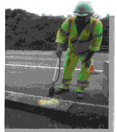
3. Place largest round piece of super bundy and apply heat. The material will start to bubble, go slightly darker in colour and the edges should fall onto the surface. NOTE "Slow Cook" the material with the burner by holding the burner slightly higher and keep moving constantly. DON'T heat too intensely.
