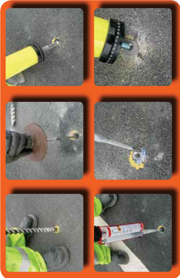
Installing an NSE Pole Cone
