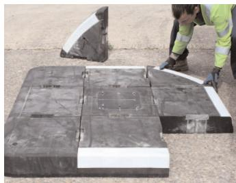
**3.** Ensure all module butt joints are tightly together and start from the middle sections of the RediPave. With a 14mm drill bit, drill through the holes to a depth of 270mm from module surface into the road. The drill used will be a Hilti T15 or T21 hammer drill (or similar) attached to a 3 kva generator via a 25 m. 110 v extension lead.
