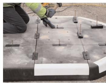
**5.** Insert coach screw through black plastic anchor block and attach Rediplug and tap down to surface level. Tighten with impact wrench; ensuring coach screw is firmly seated.
