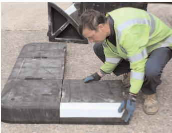
**2.** Mark position on road for location of Islands and assemble the RediPave modules accordingly.
