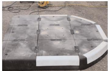
**6.** Repeat drilling, blowing, resin for remaining middle holes and use the black plastic anchor fixings to secure island. Once middle sections have been completed, drill remaining outside holes and blow out fixings holes using the long nosed air gun. Thoroughly blow out holes and insert resin commencing at base of hole, 2 to 3 pumps required.
