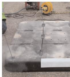
**7.** Insert coach screw and plastic washer into Rediplug. Tap assembly down to 70mm above module surface and tighten with impact wrench, ensuring washer is firmly seated.
