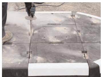
**4.** Blow out fixing holes using a long nosed air gun, powered by a 120psi portable compressor, insert resin commencing at base of hole, 2 to 3 pumps required using a resin gun supplied by Rediweld.
